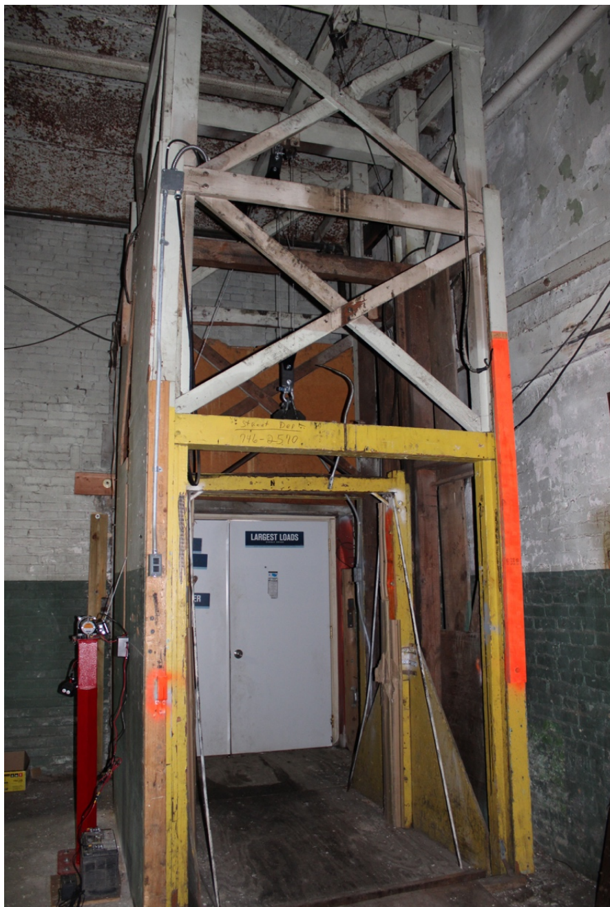
Fig. 10: Freight elevator likely installed when the building became an appliance retailer to move large appliances to and from basement storage. Photographer facing north.
