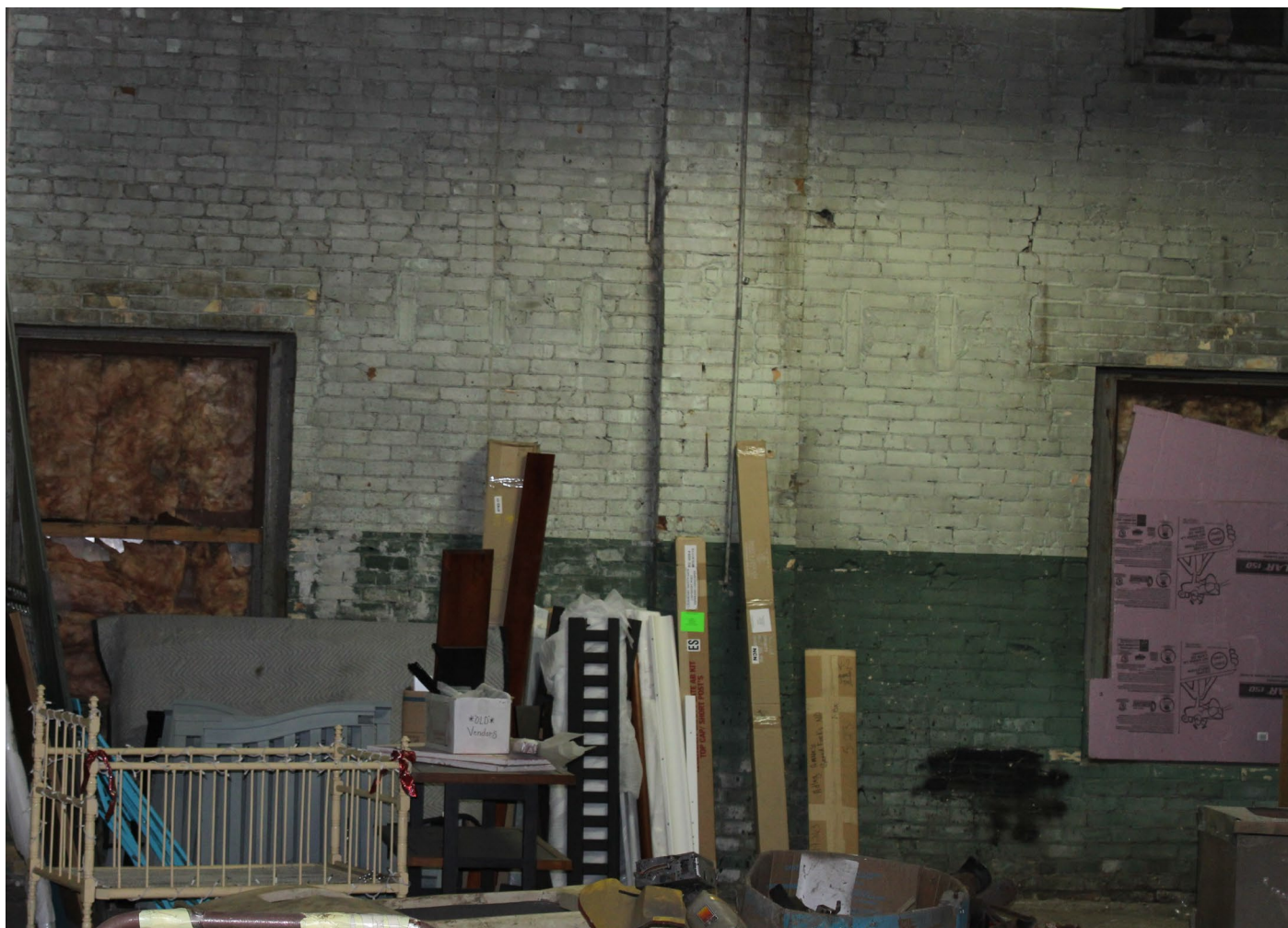
Fig. 11: Vertical scars running horizontal along the north wall approximately every 18 inches, above the green paint indicate where a spectator platform once stood. The windows along this wall (partially visible in the top right) were filled in with brick.
