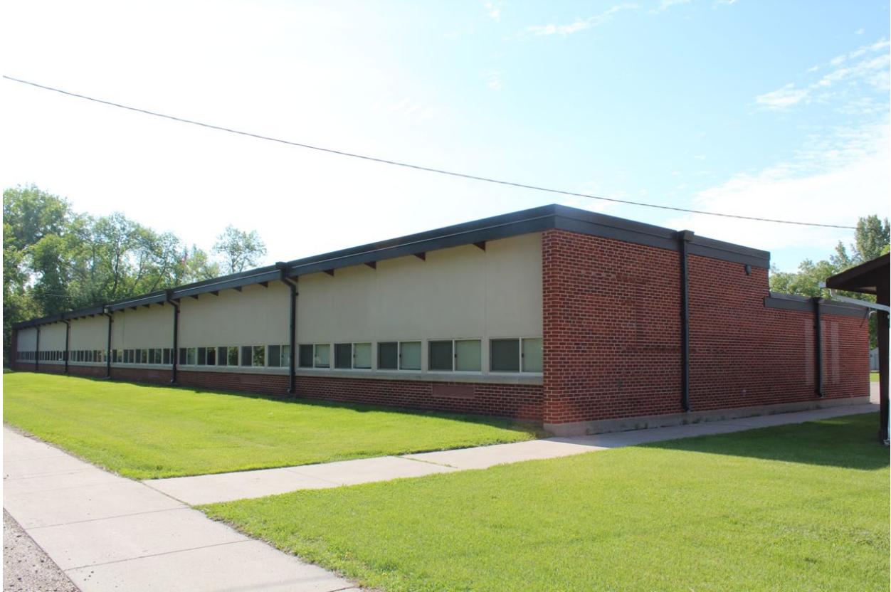
Photo 10 of 14. Digital Image: ND_Grand Forks_Grand ForksMPS_West Elementary School_0010.tiff. West elevation of north wing shows linear contemporary bond brickwork.
