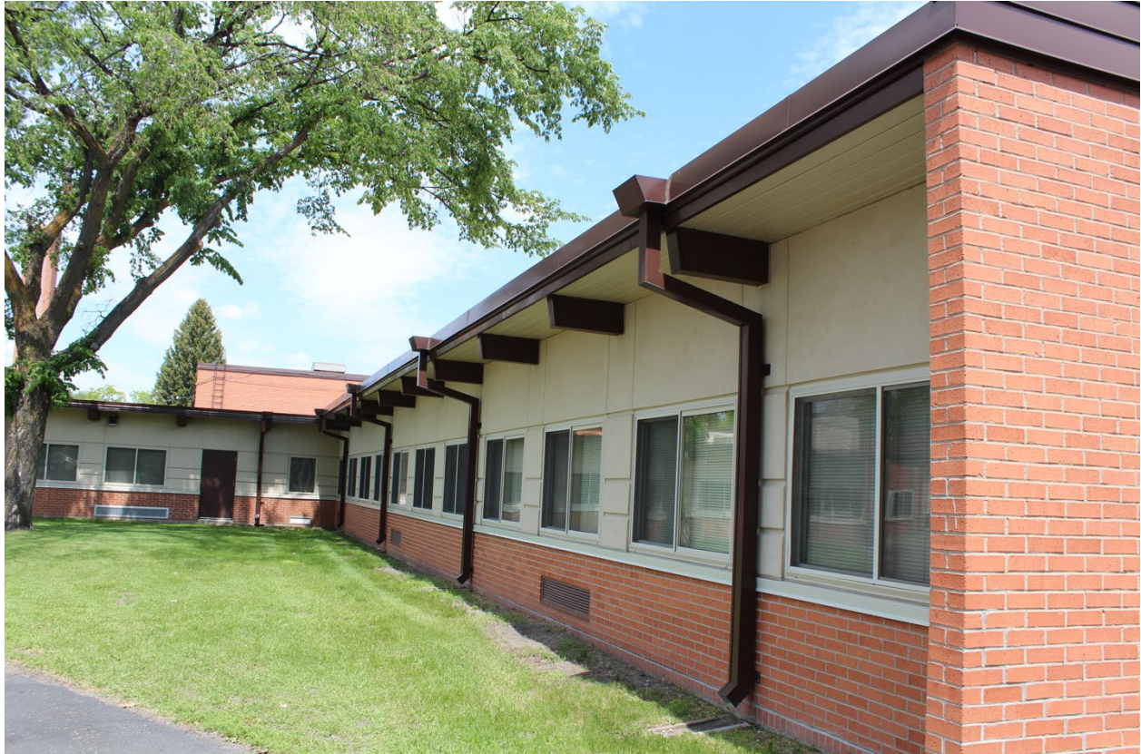
Photo 3 of 10: Digital Image: ND_Grand Forks County_Grand ForksMPS_Viking Elementary_0003.tiff. East wing showing exposed steel beams under the eaves. They extend visibly through the classrooms.
