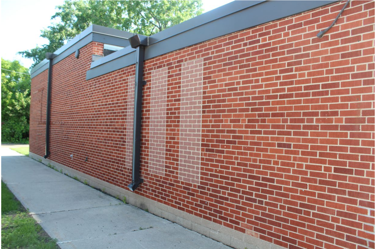
Photo 4 of 14: Digital Image: ND_Grand Forks_Grand ForksMPS_West Elementary School_0004.tiff. West elevation of north wing shows infilled windows, facing northwest.
