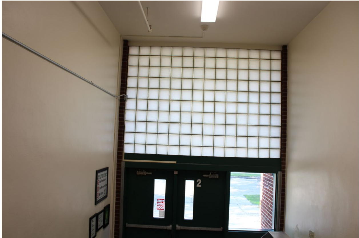
Photo 7 of 14: Digital Image: ND_Grand Forks_Grand ForksMPS_West Elementary School_0007.tiff. Glass block on the south entrance allows maximum natural light into the hallway.
