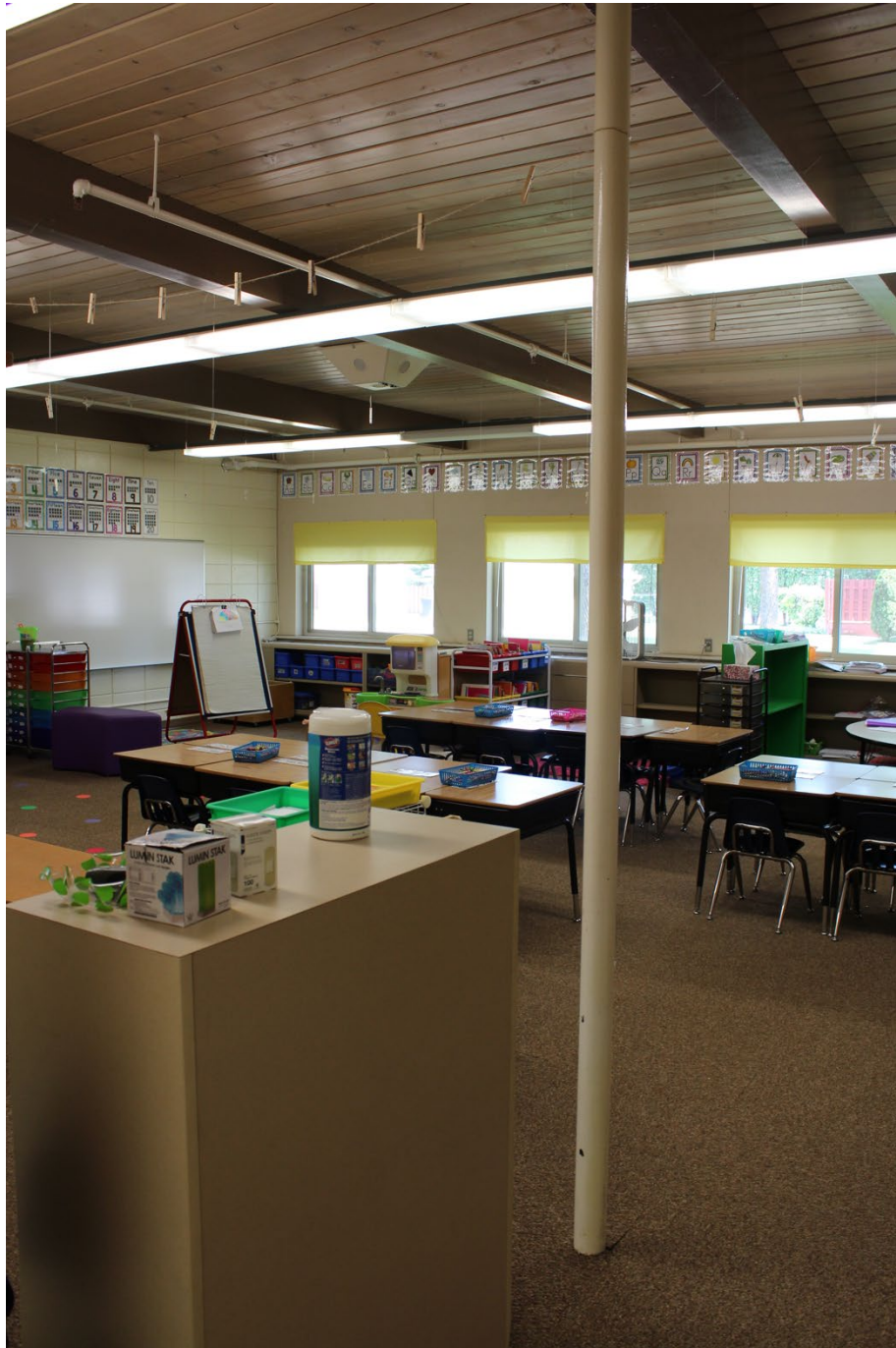
Photo 8 of 10: Digital Image: ND_Grand Forks County_Grand ForksMPS_Viking Elementary_0008.tiff. Steel posts support the exposed steel beams that run the width of the building, turning structural elements into architectural features.
