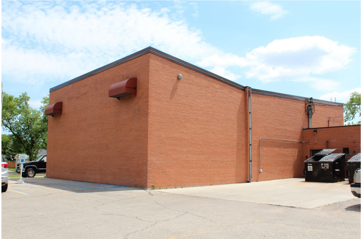
Photo 6 of 10: Digital Image: ND_Grand Forks County_Grand ForksMPS_Viking Elementary_0006.tiff. Viking gymnasium with a single pitched roof above the stage and flat roof over the remainder. Red brick is laid in a running bond both on the gymnasium and the classroom buildings.
