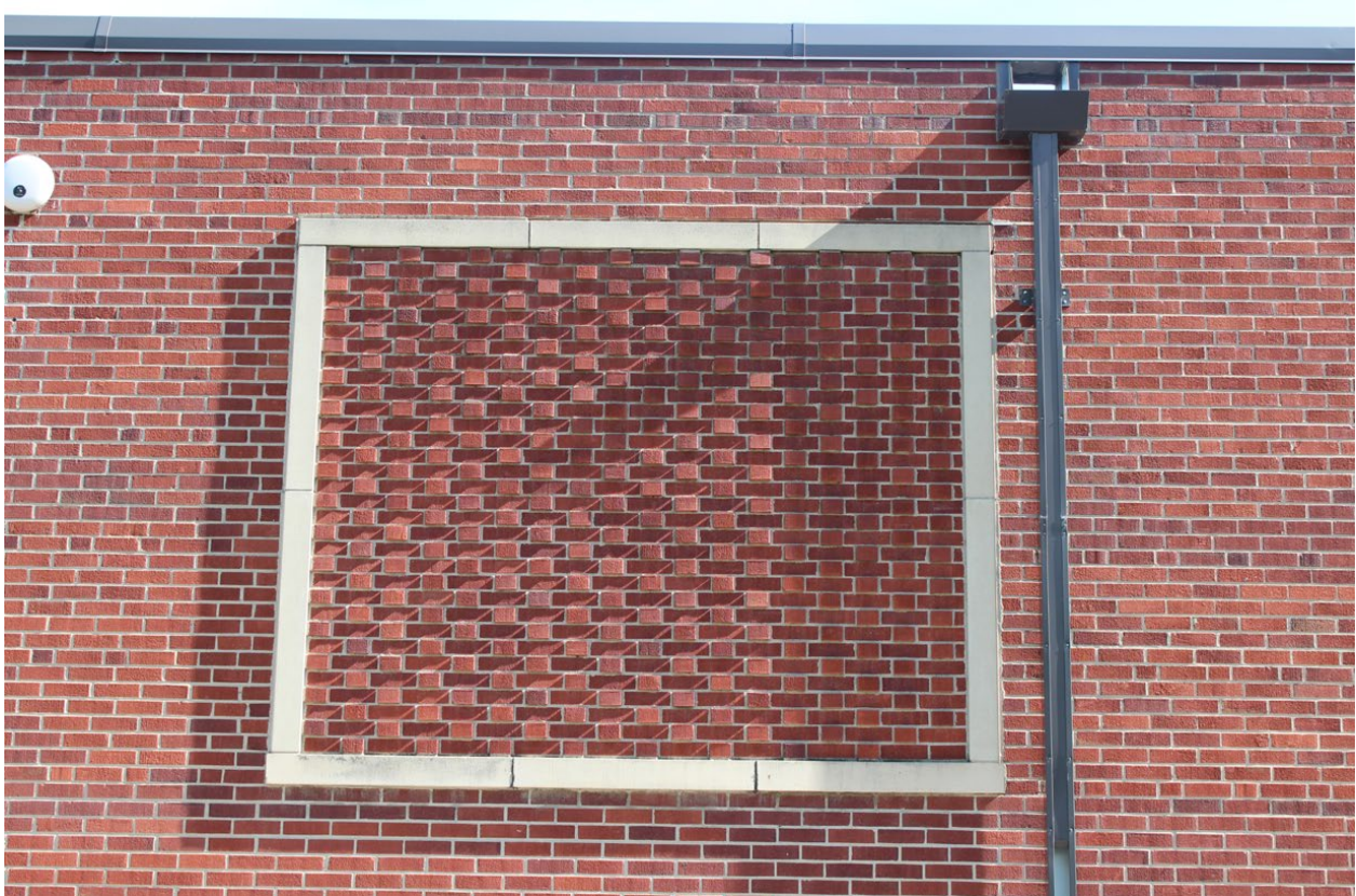
Photo 9 of 14: Digital Image: ND_Grand Forks_Grand ForksMPS_West Elementary School_0009.tiff. Decorative brick relief with a limestone frame on south elevation of east wing, facing north
