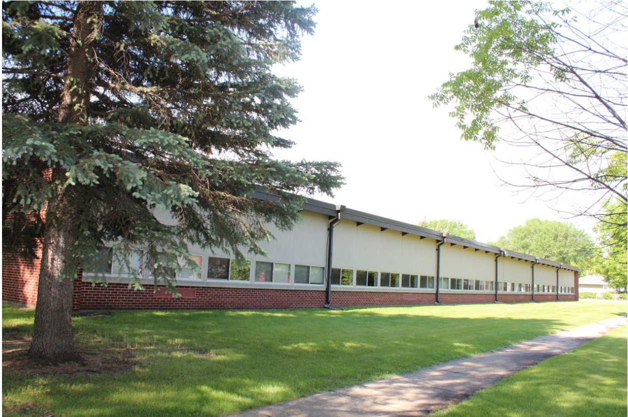
Photo 3 of 14: Digital Image: ND_Grand Forks_Grand ForksMPS_West Elementary School_0003.tiff. North elevation showing exposed steel beams extended under the eaves, facing southwest.
