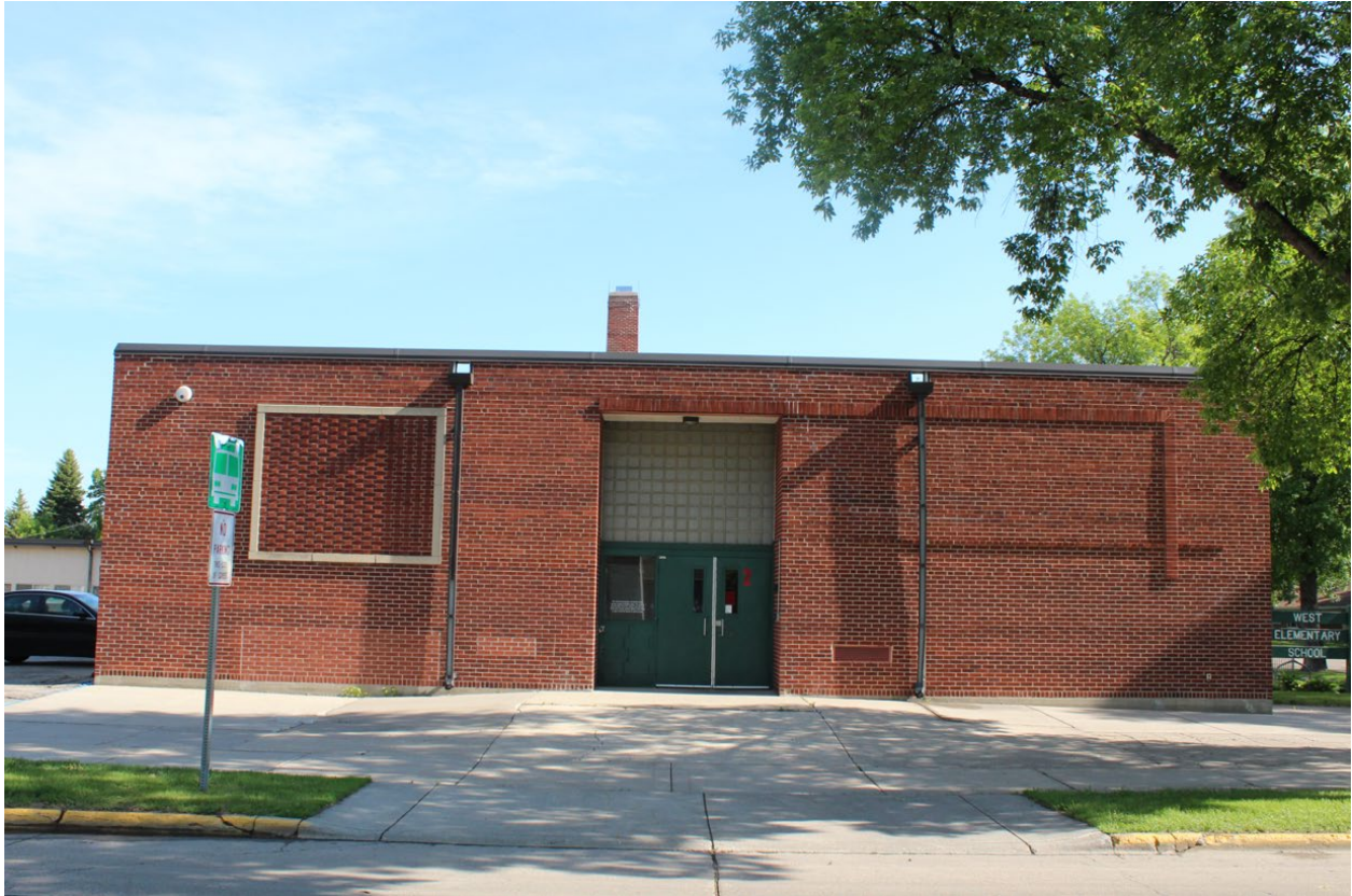
Photo 5 of 14: Digital Image: ND_Grand Forks_Grand ForksMPS_West Elementary School_0005.tiff. South elevation of east wing facing north with decorative brick relief to the left and linear contemporary bond to the right of the entrance.
