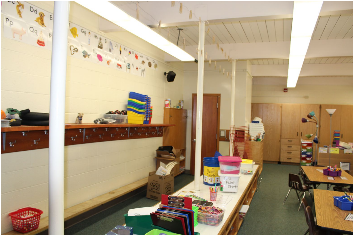
Photo 8 of 8: Digital Image: ND_Grand Forks County_Grand ForksMPS_Ben Franklin_0008.tiff. Many mid-century classrooms maintain original features such as steel posts supporting exposed steel beams, coat hooks, lots of storage for supplies, benches for project work and closets.
