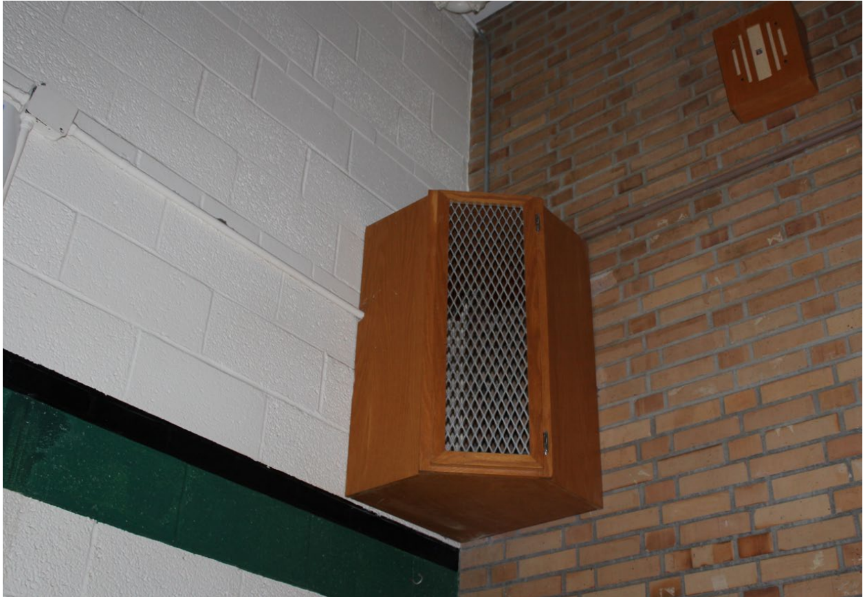
Photo 12 of 14: Digital Image: ND_Grand Forks_Grand ForksMPS_West Elementary School_0012.tiff. Exposed brick in the gymnasium in a double stretcher garden wall bond abuts the concrete block.
